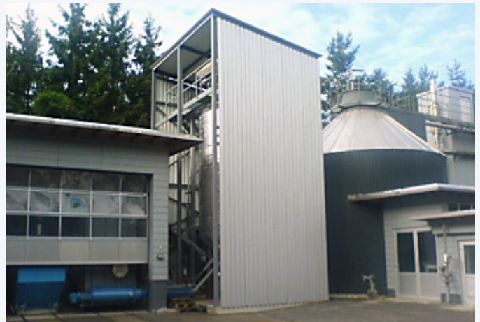
LTDry pilot plant, Switzerland
